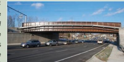
Reinvestment Act) project in CT. The objectives were to resolve the congestion issues by replacing the existing bridge and widening Route 1, as well as to address the flooding issues by adding a new culvert and reservoir.
