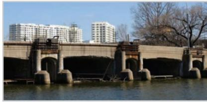
Built in 1937 and rehabilitated in 1984, Porpoise Bridge is a fourteen-span structure which carries Perimeter Road over Flushing River in the Flushing Meadows-Corona Park in Queens, NY. Perimeter Road has two lanes of traffic, one lane in each direction, with a nine-foot wide sidewalk on the south side of the structure. The bridge is approximately 37 feet wide (outside to outside) and 370 feet in length.
