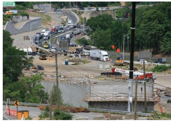
I-84 Reconstruction, Waterbury, CT
